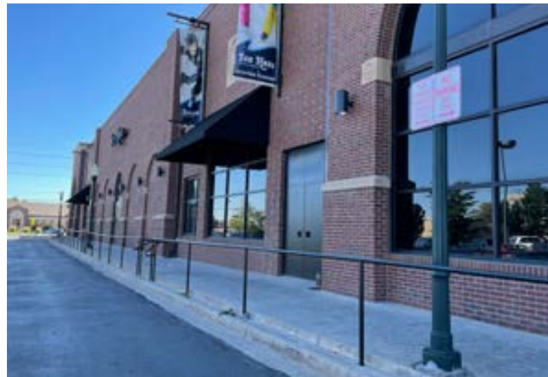
Image of the attached sidewalk and protective railing at the Greeley Ice House
