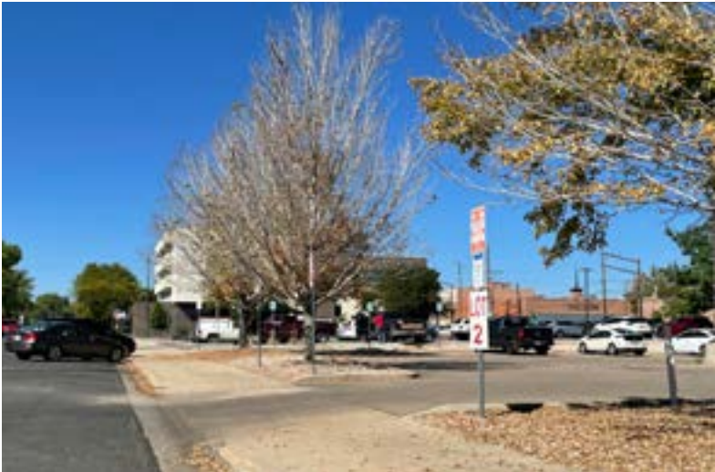
Image of an attached sidewalk next to diagonal parking
