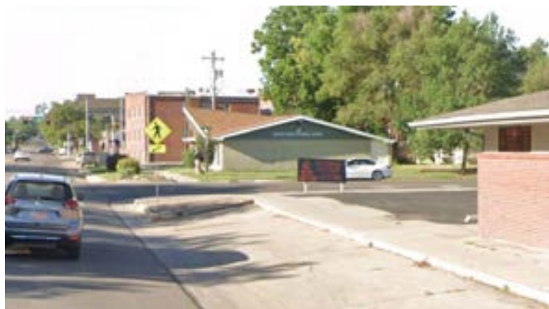
Image of blocks where the amenity area has been removed to allow for additional travel lanes and parking
