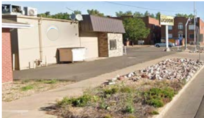
Image of a poorly maintained frontage along 11th Avenue
