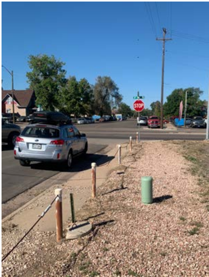
Image of dilapidated sidewalk condition on 4th Street
